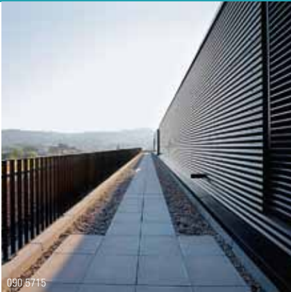
Panoramic "to-and-fro" walkway on the Cube roof, with the facade cladding the building services area
