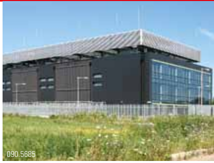
PTC data center
