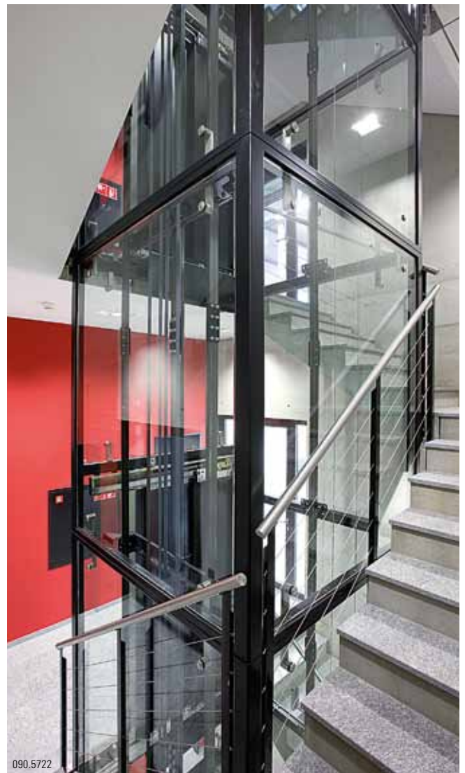
Landing in the stairway of the first floor south, with glass-surround elevator
