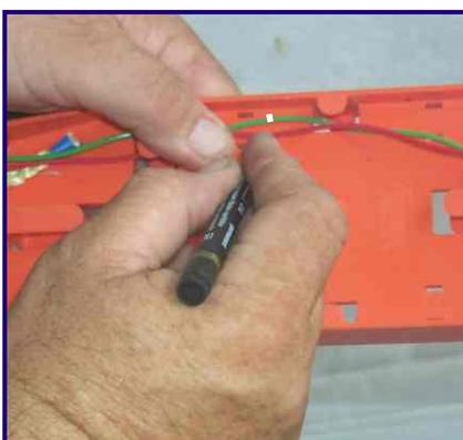
**16** Mark the fibre tubes to required length.
