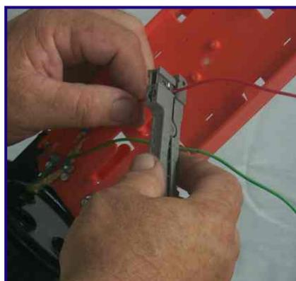
**17** Carefully remove and clean the fibre tubes as not to damage the bare fibres.
