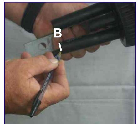
**6** Mark the cable B level with the bottom of the heatshrinkable sleeve.
